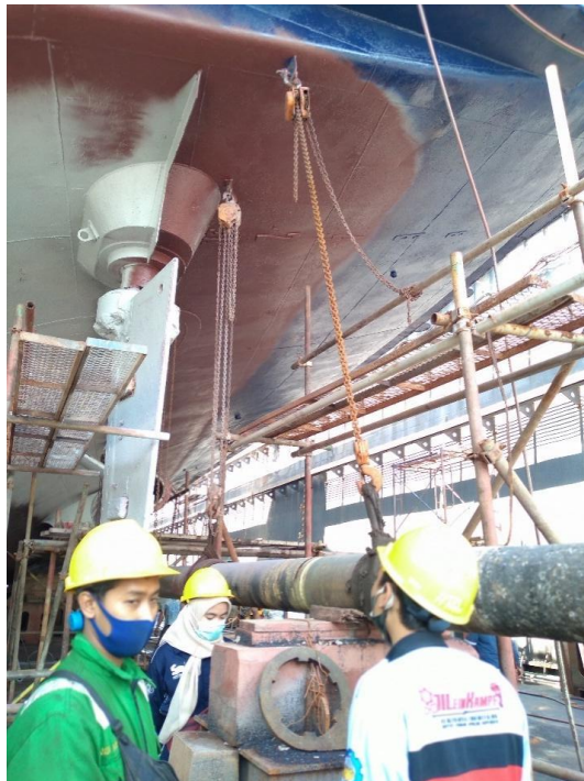
Gambar 5. 1 Scaffolding dan Chain Block
