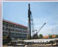
Piles Foundation for Building
