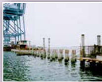
Piles for Marine Structure
