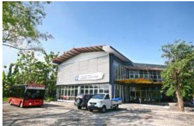
Gambar 1.4 Gedung PUI SKO & STP OTOMOTIF ITS
