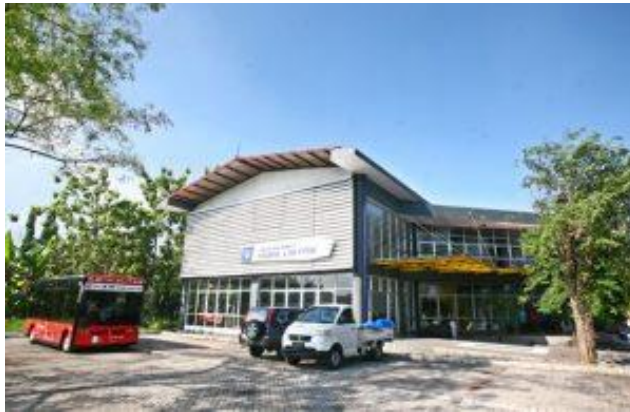
Gambar 1.4 Gedung PUI SKO & STP OTOMOTIF ITS
