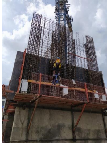
Gambar 4.54 Pemasangan Overlap Pembesian Shear Wall
