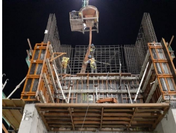
Gambar 4.59 Pengecoran Shear Wall
