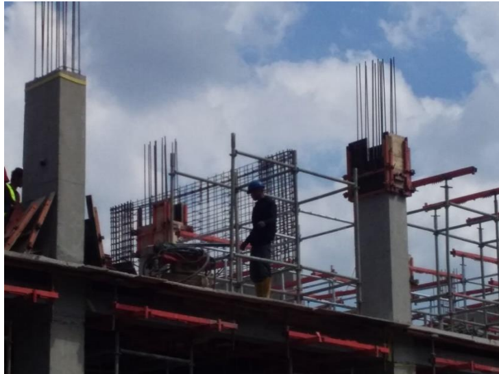
Gambar 4.31 Pemasangan Scaffolding (Four-Ways)
