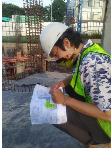
Gambar 5.7 Kegiatan Mapping Progress Bekisting, Pembesian, dan Pengecoran
