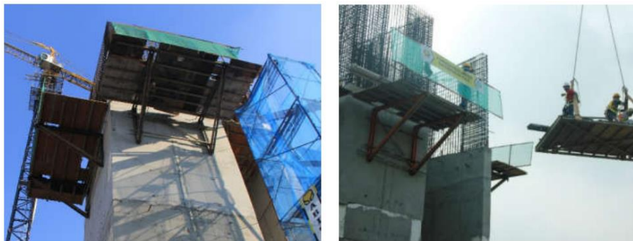
Gambar 4.53 Pemasangan Climbing Form
