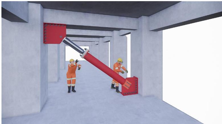
Gambar 8.7 Pemasangan Bracing HSS
