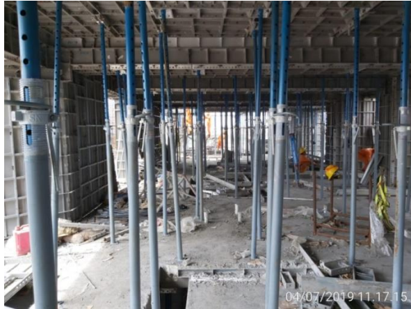
Gambar 2. 4 Metode Aluminium Formwork
