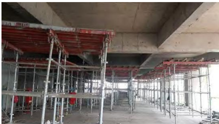
Gambar 2. 5 Metode Table Formwork Sumber: ( http://digilib.mercubuana.ac.id/ )
