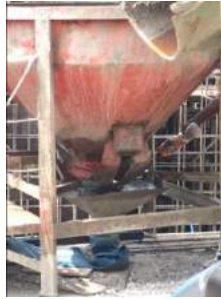
Gambar 7.11 Pemberian Solar ke Concrete Bucket
