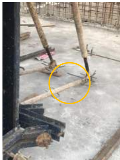
Gambar 7.5 Push Pull Bracket / Kicker Base
