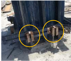
Gambar 7.2 Wedge Head Piece
