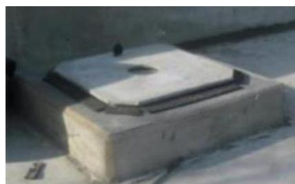
**Gambar 10-9.** Grouting Base Plate
