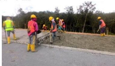
Gambar 6.8. Pekerjaan Lean Concrete
