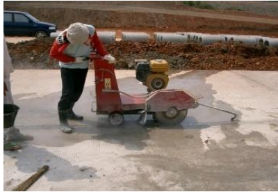
Gambar 6.15. Cutting Beton Sumber : www.google.com
