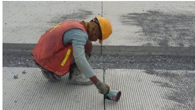
Gambar 6.16. Pengisian Joint Sealent Sumber : www.google.com
