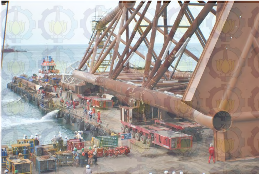
Gambar 4.16. Proses Final Completion Jacket FP-2
