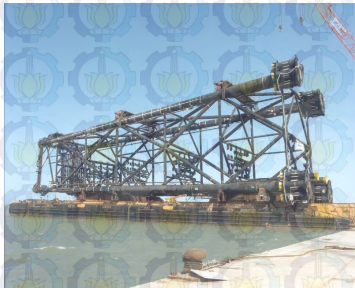
Gambar 2.1. Jacket Structure
