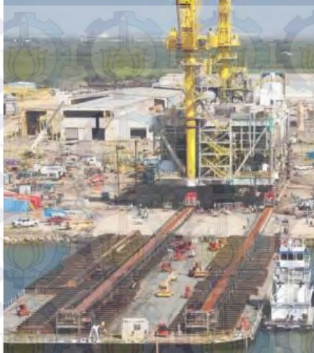
Gambar 2.3. Skidding System
