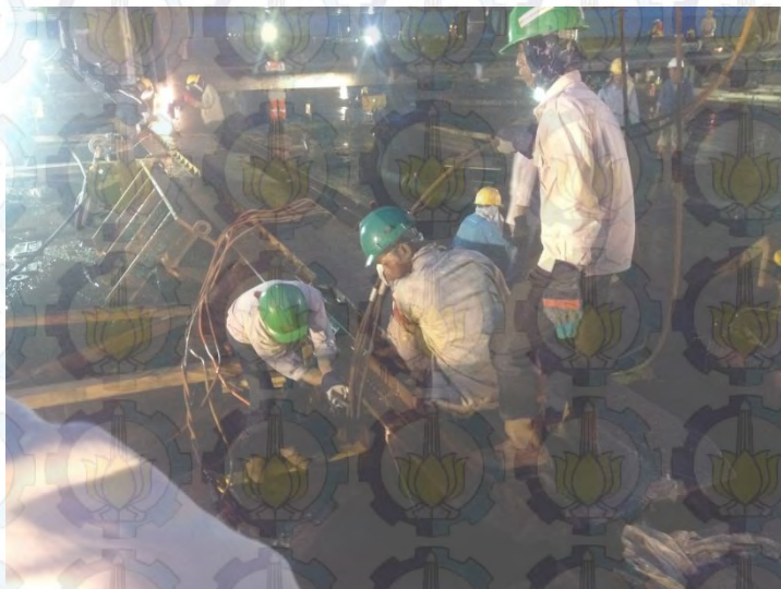
Gambar 4.12. Proses Pengelasan Grillage
