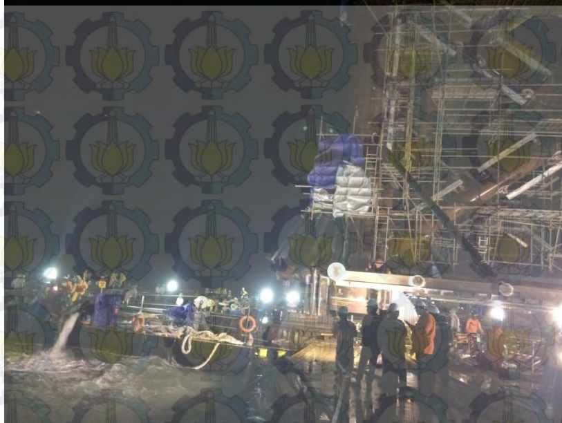
Gambar 4.7. Proses Loadout Jacket C24-P3 Sumber : (PT. XXX)
