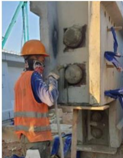
Gambar 4. 38 Pekerjaan grouting girder
