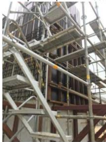
Gambar 4. 20 Bekisting pier
