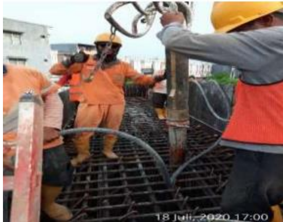
Gambar 4. 27 Pengecoran pier head
