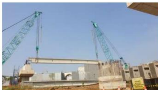
Gambar 4. 40 Proses erection girder
