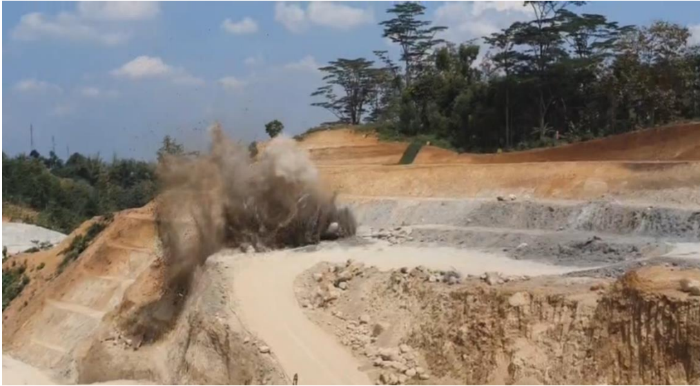
Gambar 4.19 Ledakan saat galian blasting
