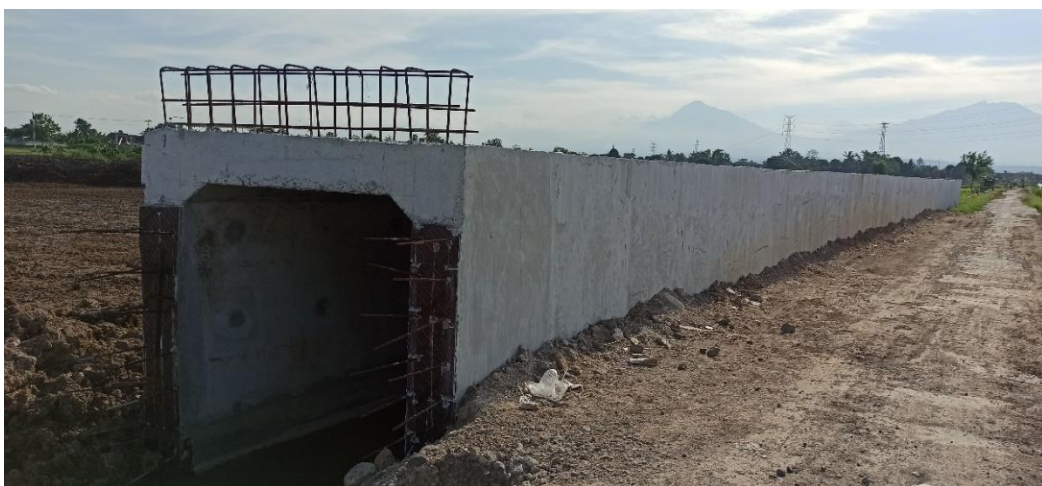
Gambar 4. 2 Box Culvert STA 0+865
