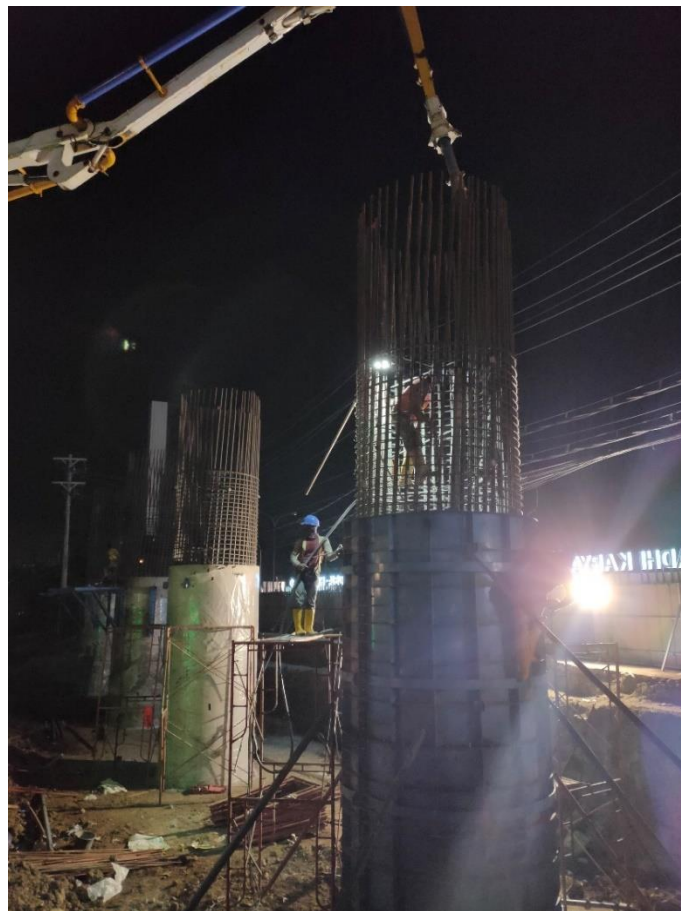
Gambar 4. 8 Pengecoran Segmen 1 Kolom Pier Underpass
