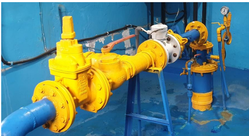
Gambar 2.4 Pompa Sistem Distribusi Sumpster
