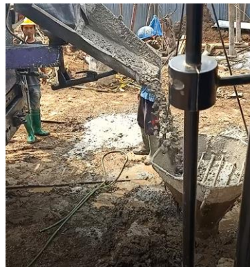
Gambar 5. 10 Pengecoran bored pile
