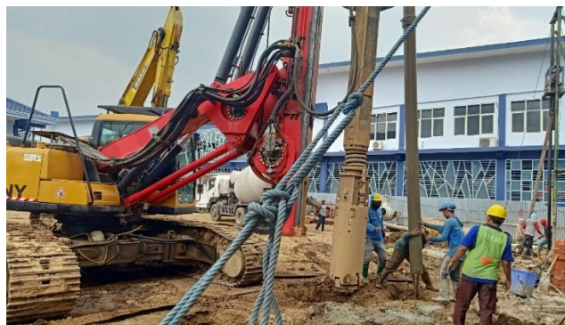
Gambar 5. 11 Pengecoran bored pile
