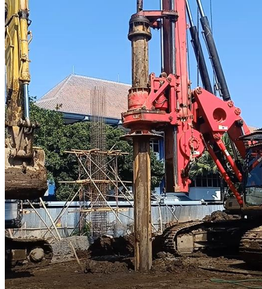
Gambar 5. 3 Pengeboran bored pile
