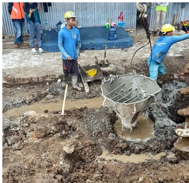
Gambar 4.9 Pengecoran bored pile
