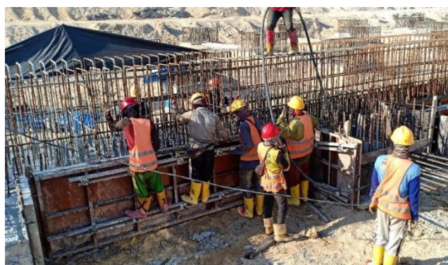
Gambar 3.3.8 Pengecoran Capping Beam Tahap 1
