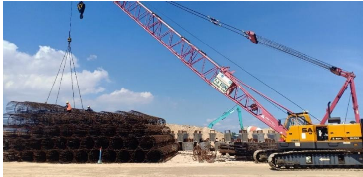
Gambar 3.1.9 Lifting Tulangan Borepile
