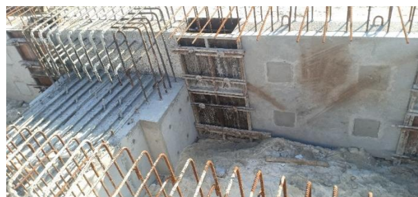
Gambar 3.3.29 Instalasi Bekisting Joint Lisplank
