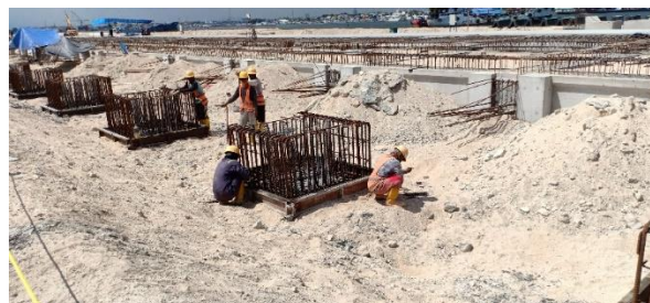
Gambar 3.3. 46 Instalasi Tulangan Joint Beam
