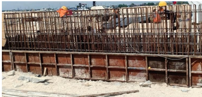
Gambar 3.3.7 Pekerjaan Bekisting Capping Beam
