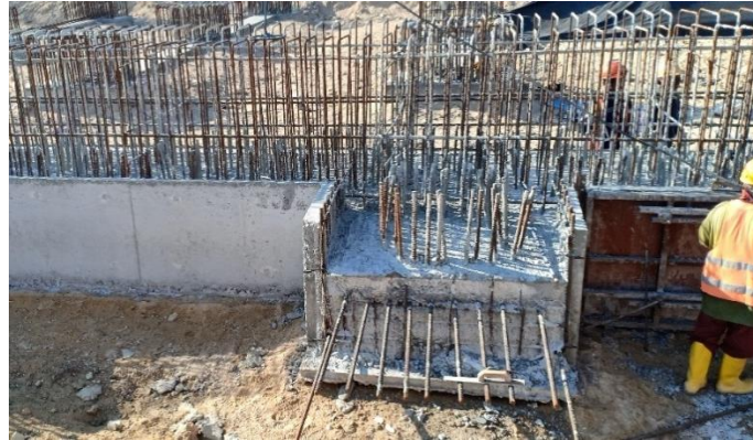
Gambar 3.3.9 Tampak Capping Beam tahap 1
