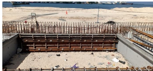
Gambar 3.3.22 Bekisting Capping Beam tahap 2
