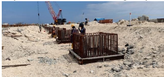
Gambar 3.3. 48 Instalasi Bekistin Joint Beam
