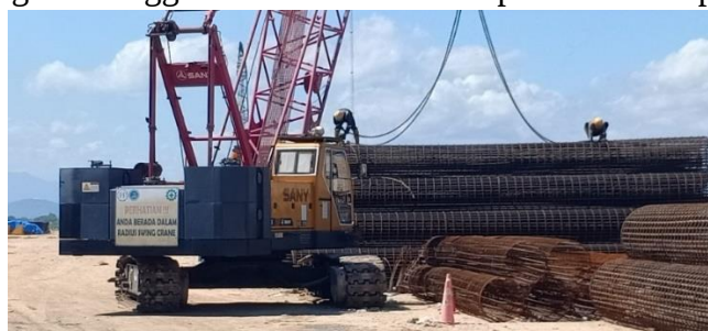
Gambar 3.1. 24 Lifting tulangan Borepile
