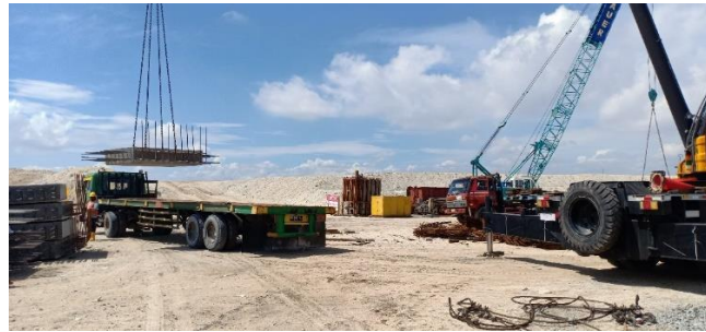
Gambar Lifting Precast Panel Plat
