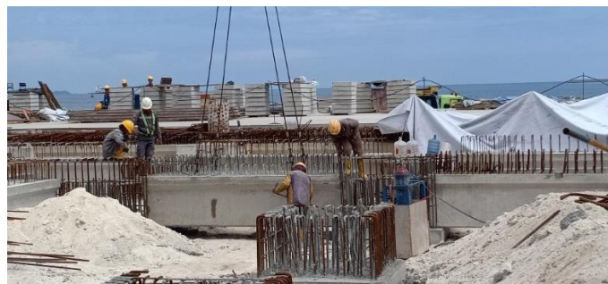
Gambar 3.3. 54 Instalasi Long Beam
