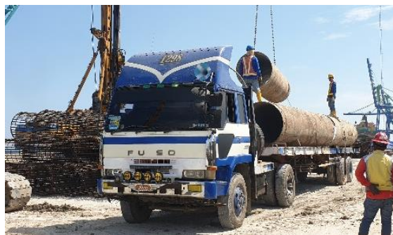
Gambar 3.1.5 Lifting Casing Bor
