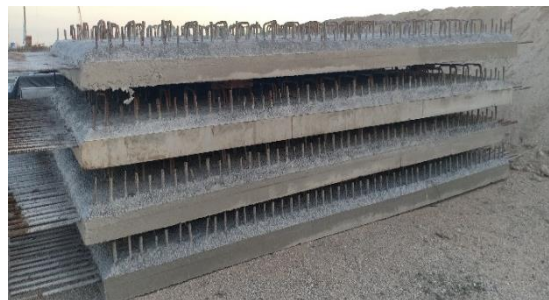
Panel Precast disimpan sementara di Storage Area
