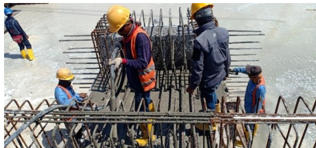
Gambar 3.3.20 Pengecoran Plank Fender
