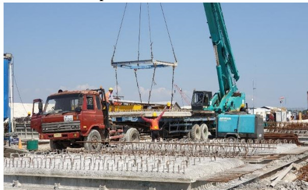
Lifting Panel Plat Precast
