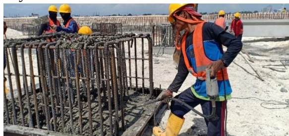
Gambar 3.3. 49 Pengecoran Joint Beam 20 cm
