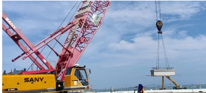
Gambar 3.3. 52 Lifting Long Beam
