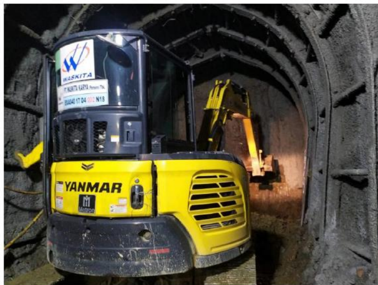
Gambar 3. 10 Scaling Hasil Galian Tunnel
