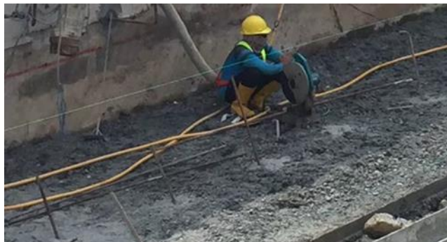
Gambar 4. 4 Lean Concrete dan Angkur
