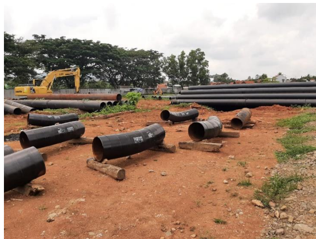
Gambar 2.9 Site Office (Area Bending)
