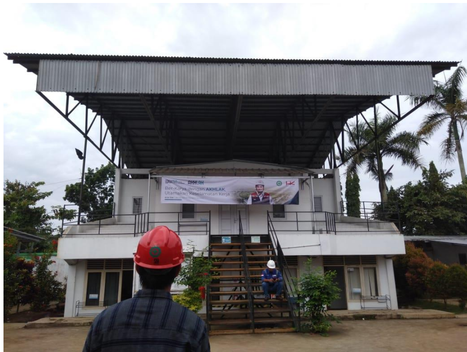
Gambar 2.3 Site Office (Ruang Meeting, Divisi Engineering , dan Divisi Legal)
