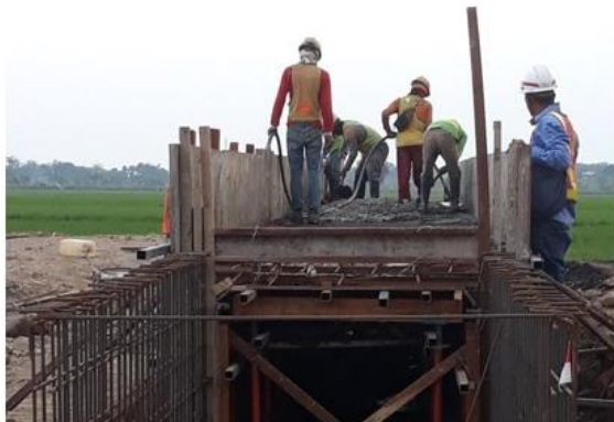
Gambar 3. 28 Pengecoran Box Culvert
