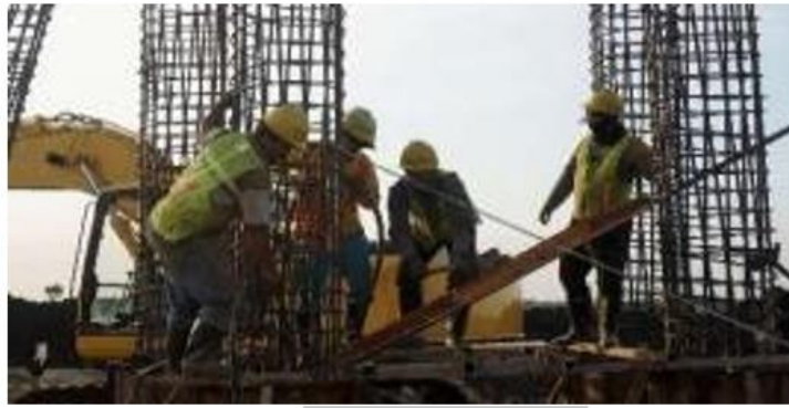
Gambar 3. 21 Proses Pengecoran Bored Pile
