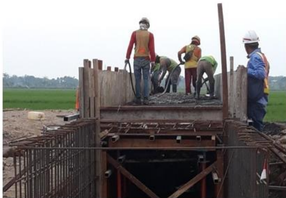
Gambar 3. 28 Pengecoran Box Culvert
