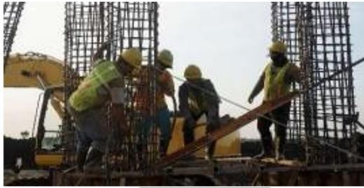
Gambar 3. 21 Proses Pengecoran Bored Pile
