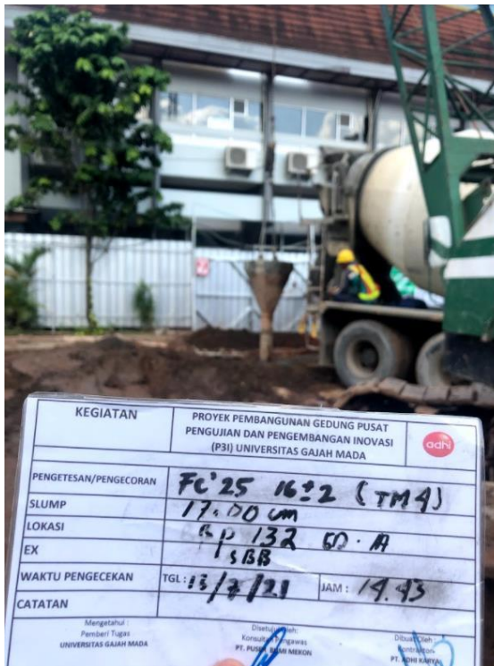
Gambar 5. 8 Proses pengecoran bore pile
