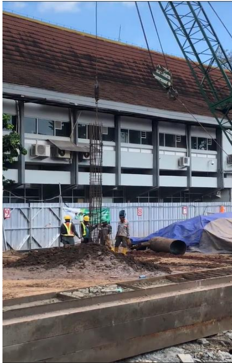
Gambar 5. 7 Instalasi Tulangan Bore pile
