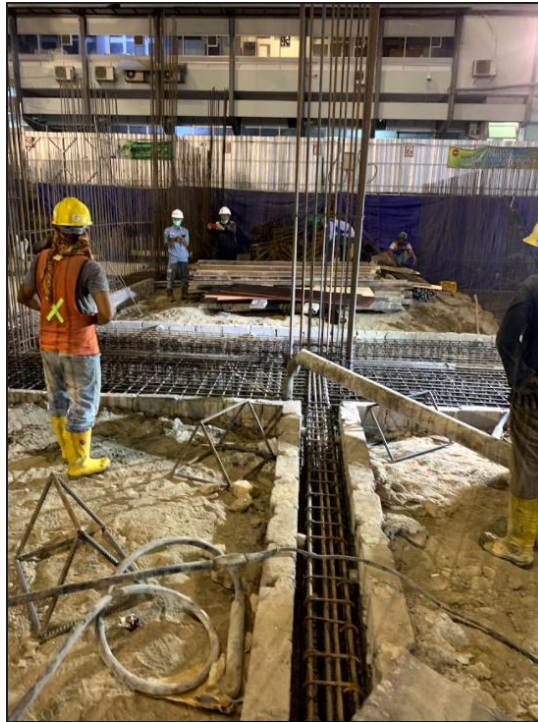
Gambar 4. 19 Pengecoran Tie Beam
