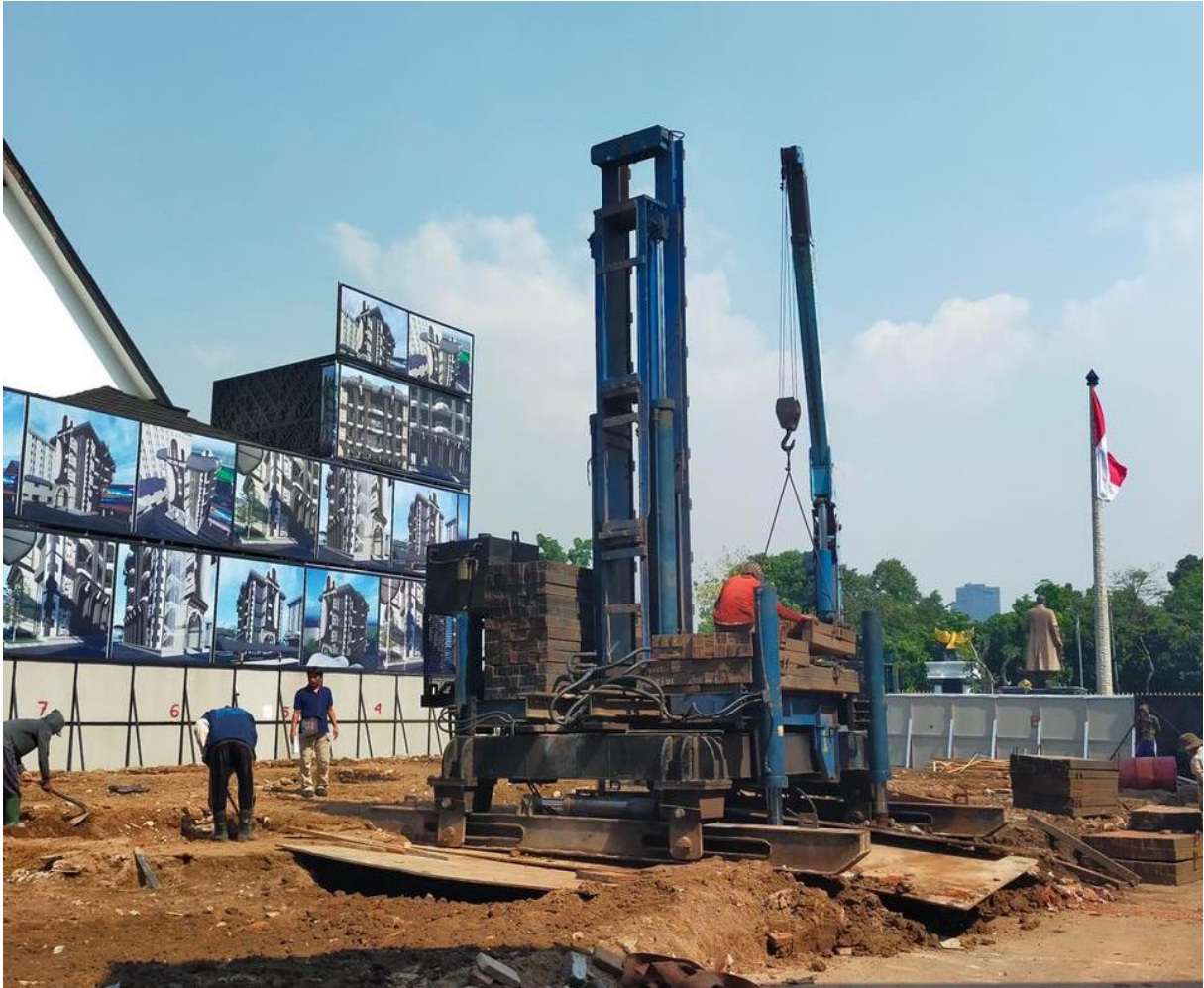
Gambar 3.5 Proses setting alat Hydraulic Static Pile Driver
