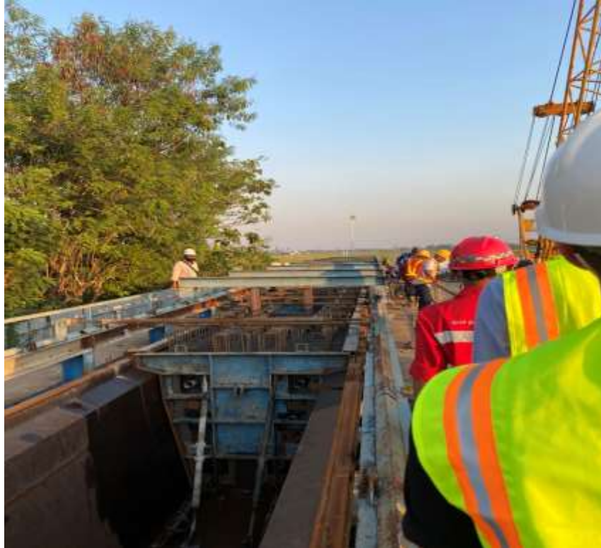
Gambar 2. 32. Proses Percetakan Girder di Batching Plant Abipraya Beton
