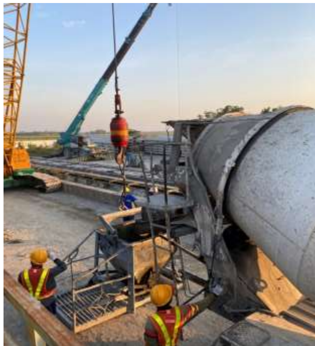
Gambar 2. 31. Proses Pengcoran Girder di Batching Plant Abipraya Beton
