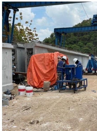
Gambar 3. 34 Proses Setting Mesin Grout Pump
