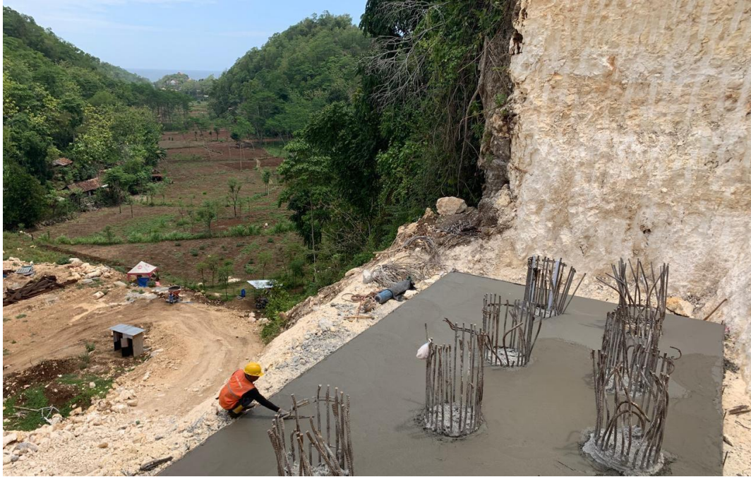
Pekerjaan Plat Lantai Abutment 1 STA 8+550
