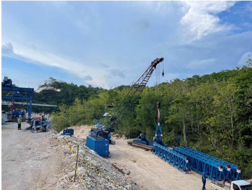
Gambar 3. 44 Proses Setting Peralatan Portal Gantry
