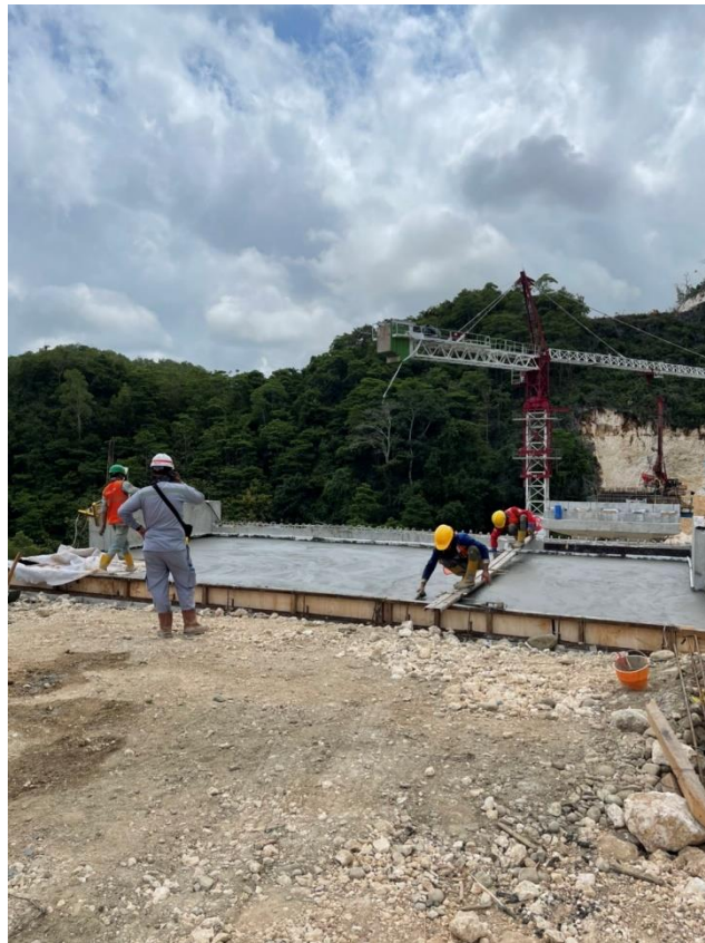
Pekerjaan Plat Lantai Abutment 2 STA 8+650
