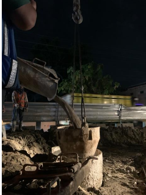
Gambar 3. 42 Proses pengecoran bored pile
