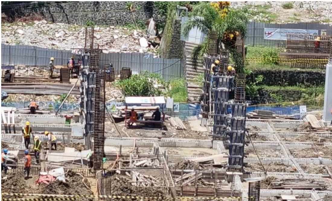
Gambar 4.45. Monitoring progress tie beam (Sumber : Dokumentasi pribadi)
