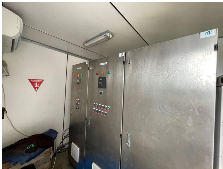
Fig. 3. 4 Capacitor bank 500kvar 12 step
