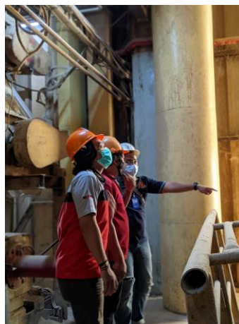
Gambar 35 Checking Screw Conveyor
