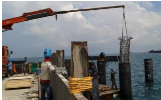
Gambar 3.5 Instalasi Besi PHT
