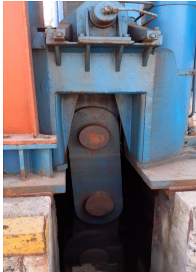
Gambar 4.1 Kondisi chain saat platform dinaikkan
