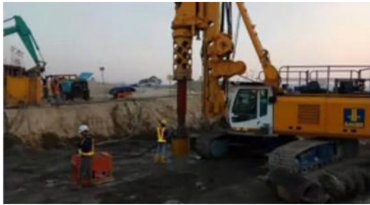
Gambar 2. 11 Proses Boring Secant Pile
