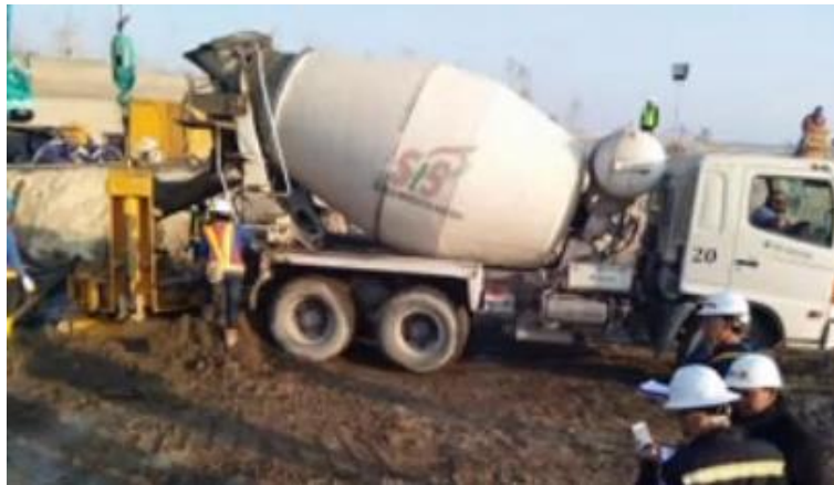
Gambar 2. 12 Proses Puring Concrete Secant Pile
