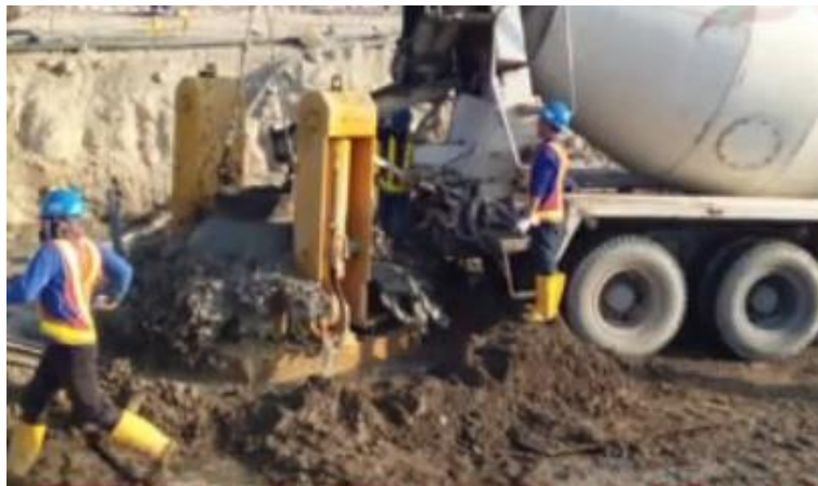
Gambar 2. 13 Proses Overtop Concrete Secant Pile
