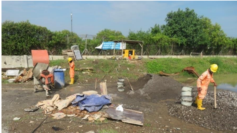
Gambar 3.10 Proses Penampuran Material Beton
