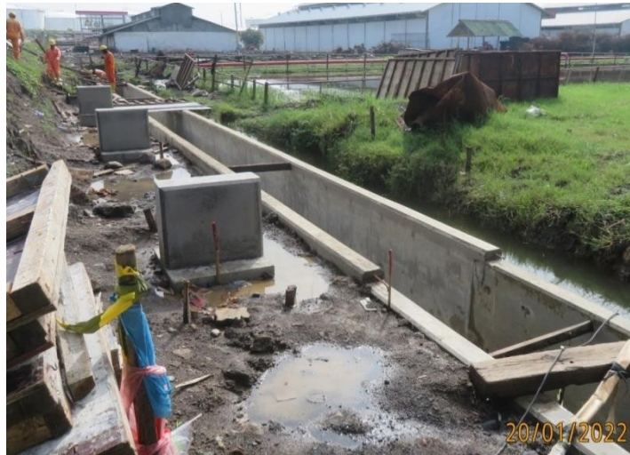
Gambar 3.23 Pipe Support Selesai Di Cor
