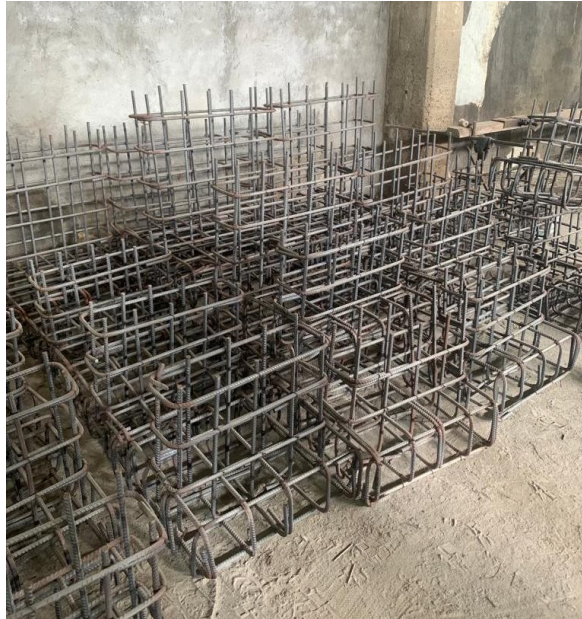
Gambar 3.20 Tulangan Pipe Support
