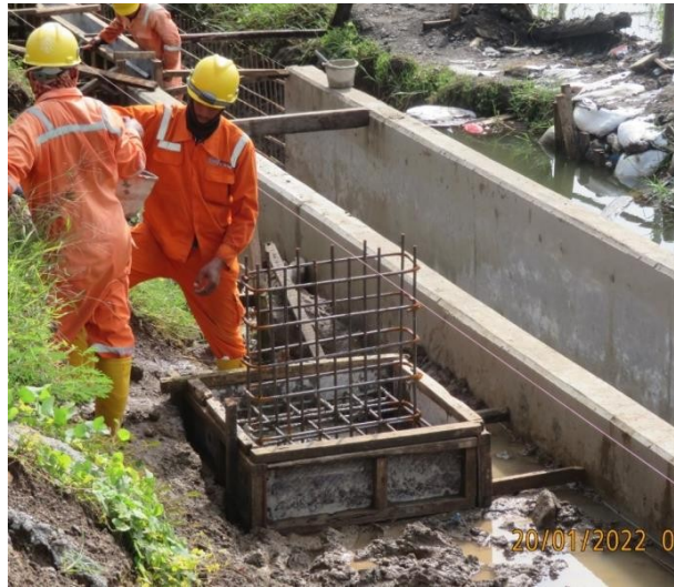
Gambar 3.22 Pengecoran Pipe Support
