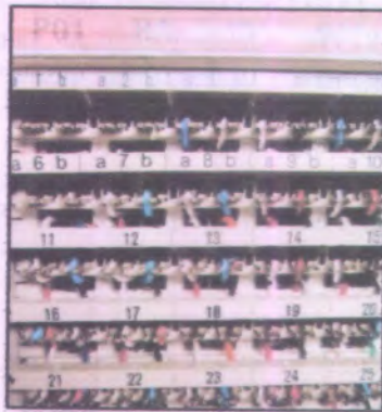
Gambar 4.11 Nomor-nomor Kabel didalam MDF
