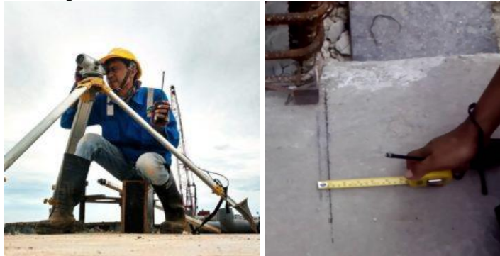
Gambar 3.24 Surveying as kolom
