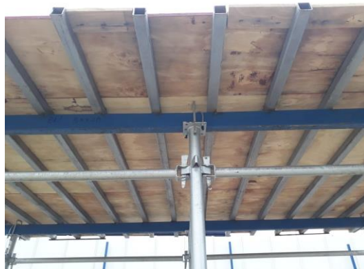
Gambar 3.5 Pemasangan primary beam, hollow, dan multiplek
