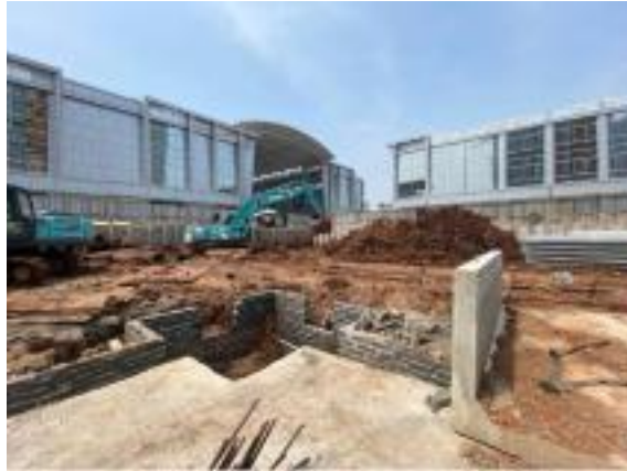
Gambar 2.14 Bekisting Batu Bata
