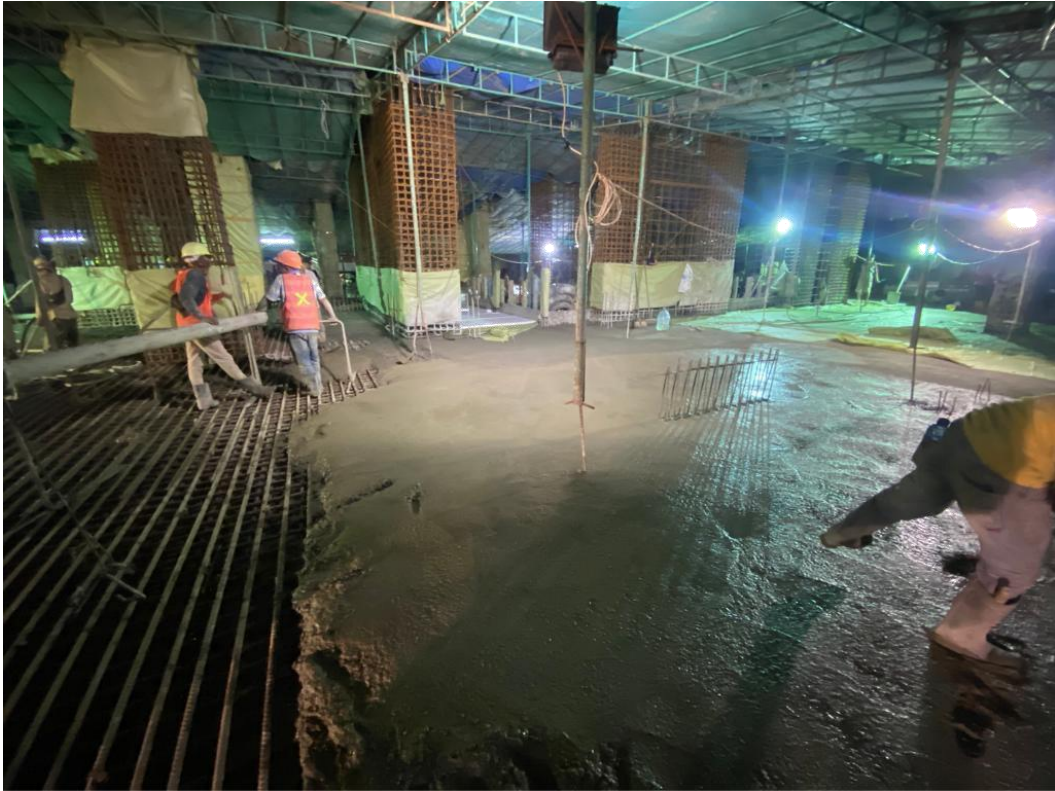
Gambar 4.12 Foto Pengecoran Raft Foundation Tower 9 Saat Malam Hari
