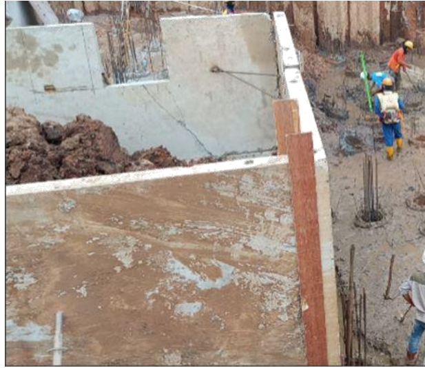
Gambar 2.16 Bekisting L-Shape
