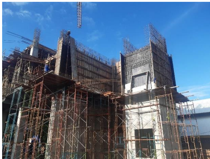
Gambar 3.18 Pekerjaan Bekisting Shear Wall
