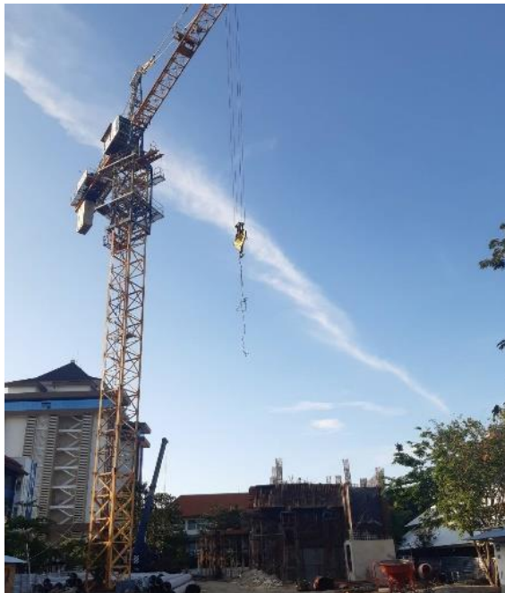
Gambar 3.33 Tower Crane Proyek
