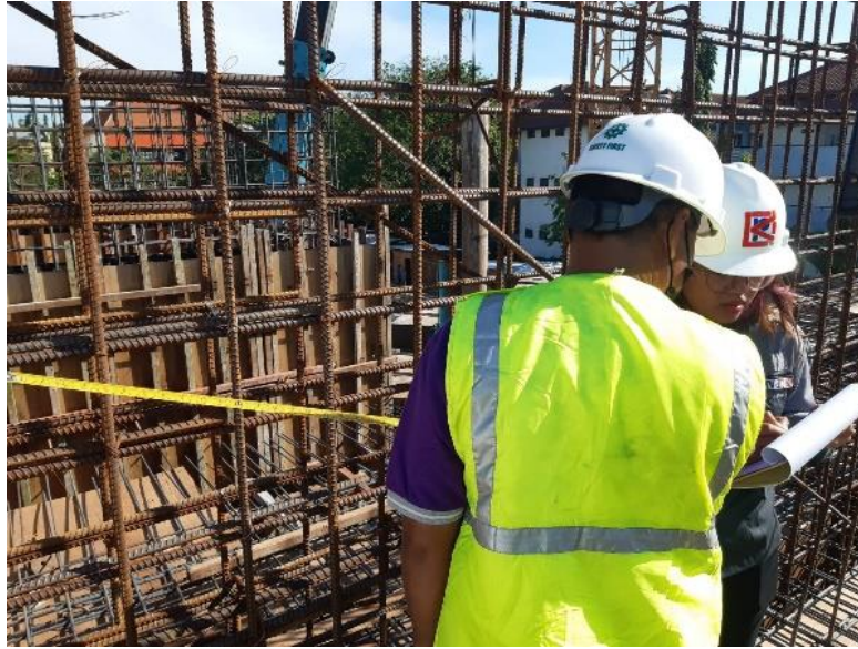
Gambar 4.2 Pengecekan Check List Pengecoran
