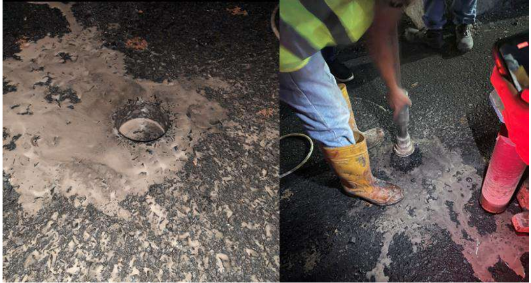
Gambar 3. 42 Pengeboran Core Drill
