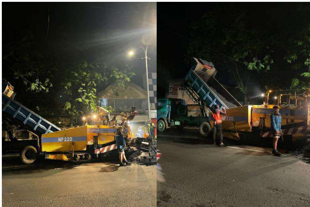
Gambar 3. 17 Proses Penghamparan Aspal
