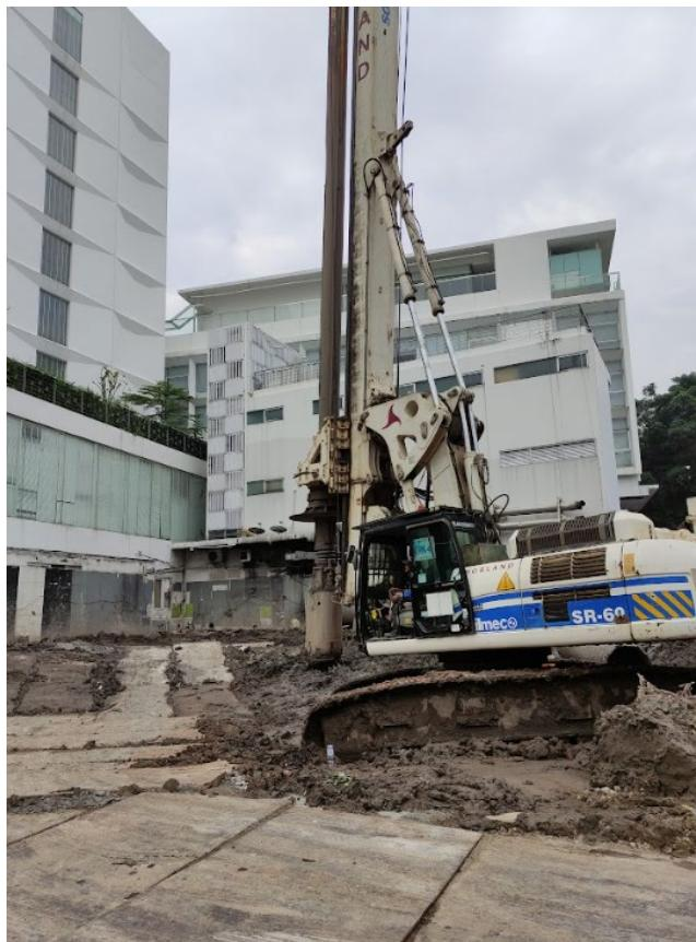
**Gambar 4.20** Mesin bor Soilmec Hydraulic Rotary Rig-SR-60
