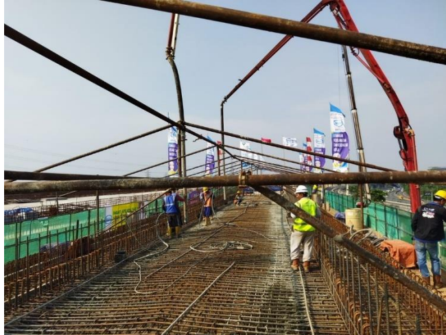
Gambar 4. 14 Proses pengecoran box girder
