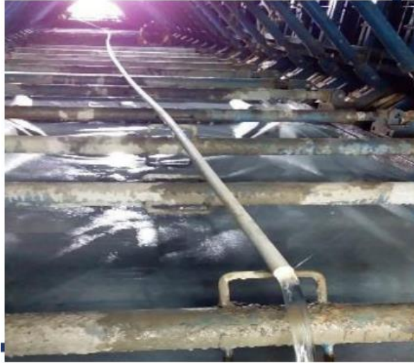
Gambar 4. 18 Proses perawatan beton didalam box girder
