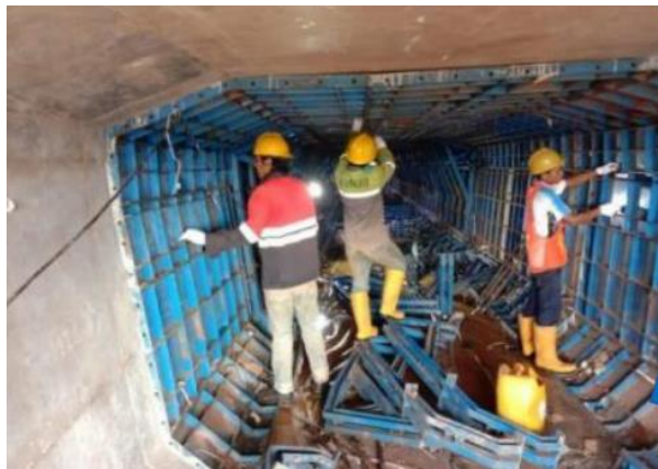
Gambar 4. 19 Proses pelepasan bekisting inner
