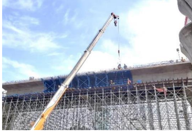
Gambar 4. 20 Proses pelepasan bekisting outer
