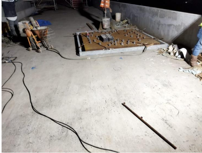
Gambar 4. 42 Proses grouting baseplate
