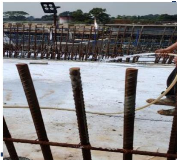
Gambar 4. 17 Proses perawatan beton diatas box girder
