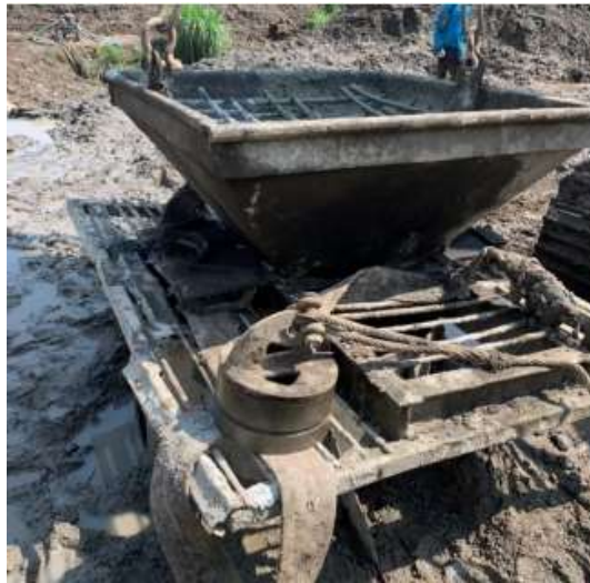
Gambar 2.13 Pengecoran Tiang Bore Pile
