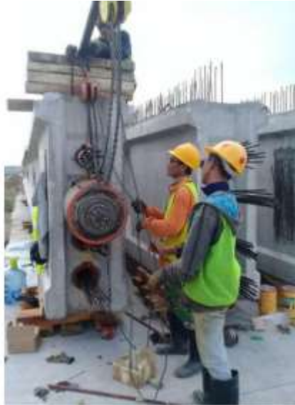
Gambar 2.23 Pelaksanaan Stressing Girder
