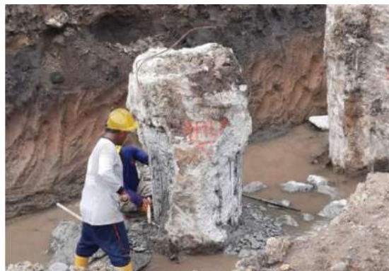
Gambar 2.26 Proses Pembobokan Tiang Bore Pile
