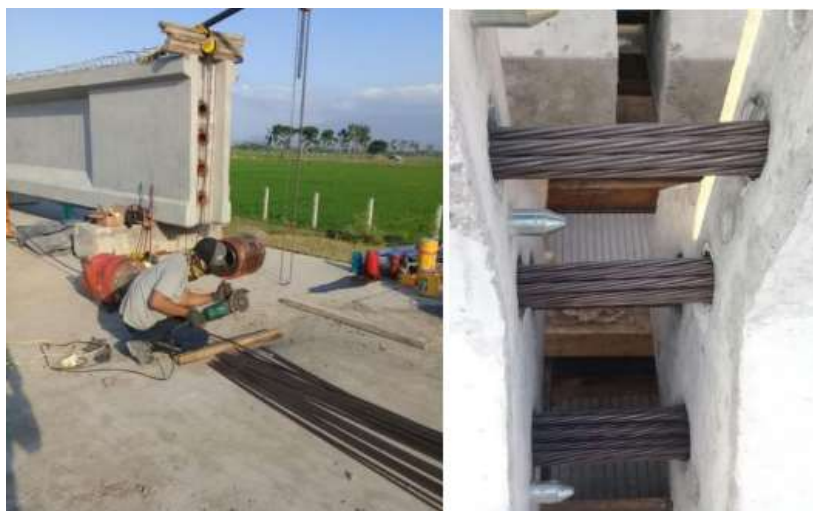
Gambar 2.20 Strand PCI Girder
