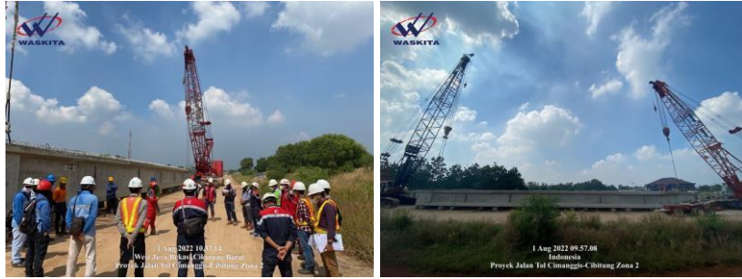
Gambar 3. 18 Load Test di Stock Yard
