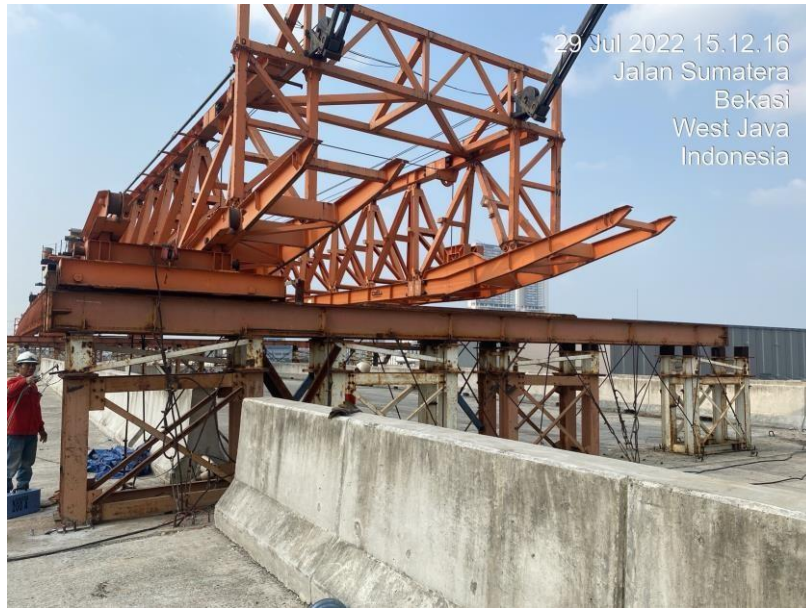
Gambar 3. 3 Rail and Roller Assembly
