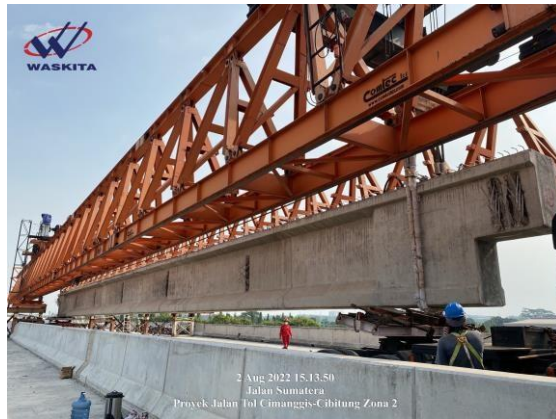
Gambar 3. 24 Lifting Girder
