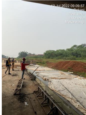
Gambar 2. 5 Proses Curing Beton
