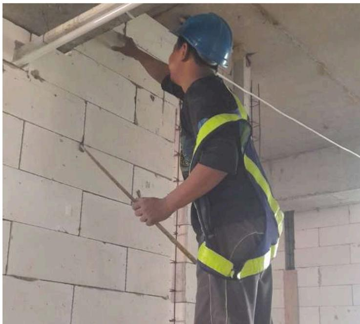
Gambar 3. 7 Pemasangan Dinding Bata
