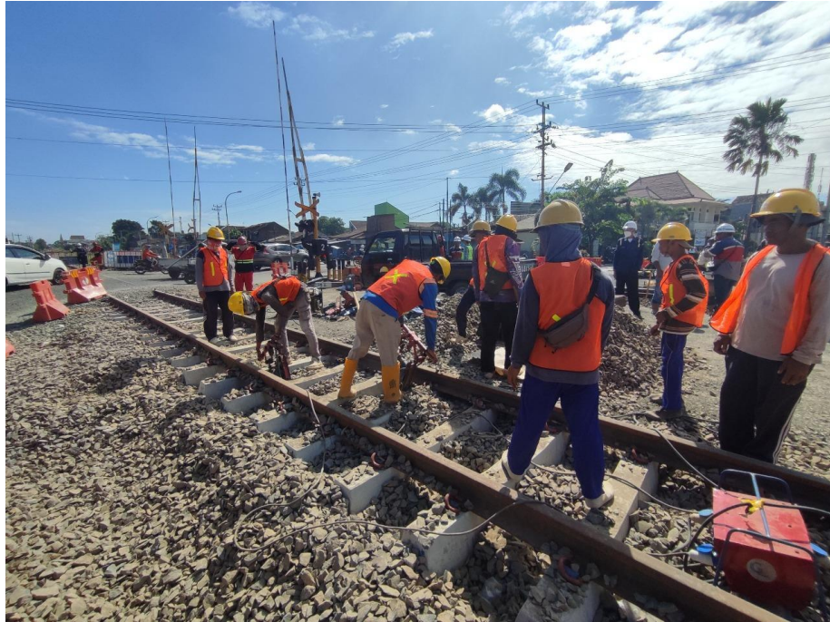
Gambar 2. 11 Proses Profiling Ballast
