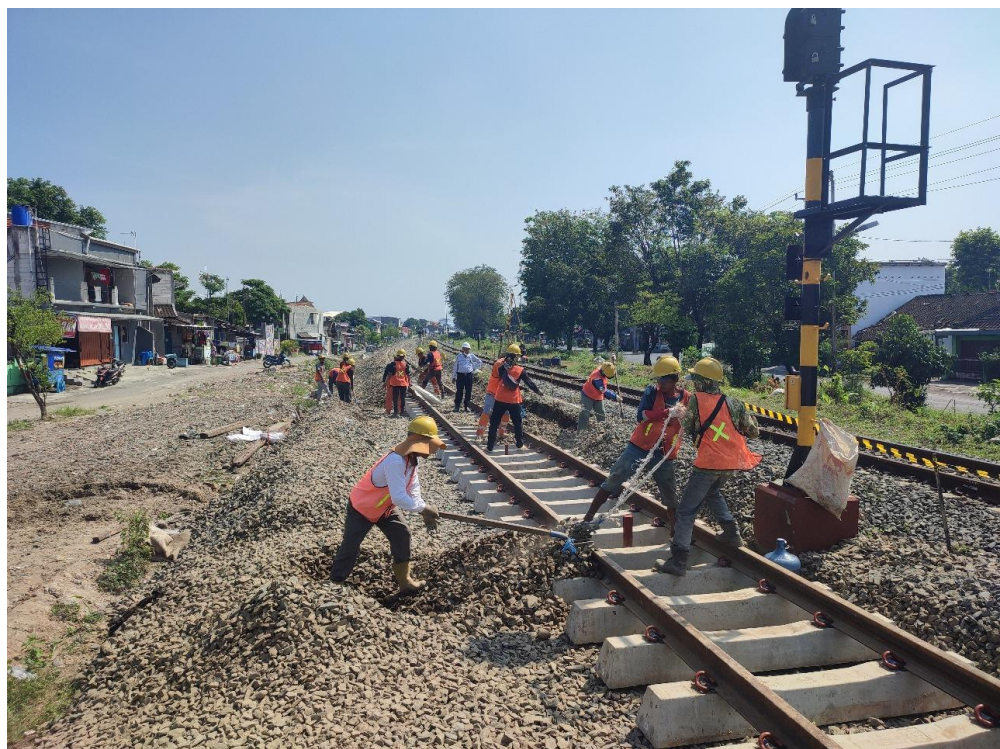
Gambar 14 Proses Profiling Ballast
