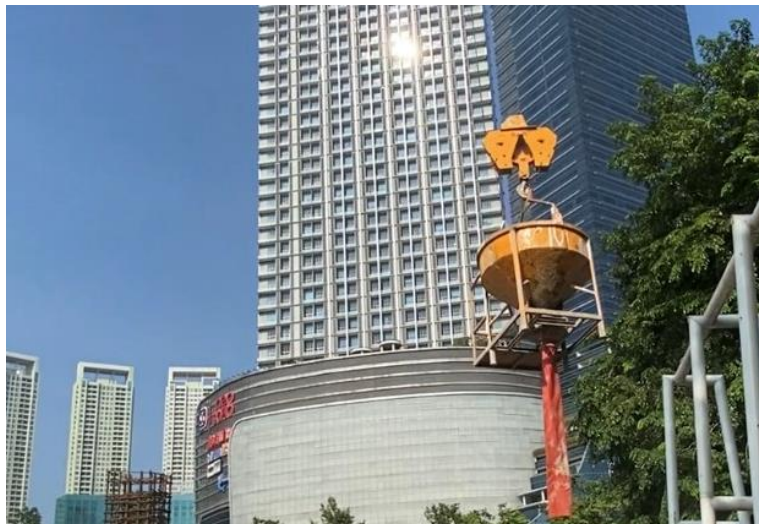
Gambar 17. Concrete Bucket dan Pipa Tremie
