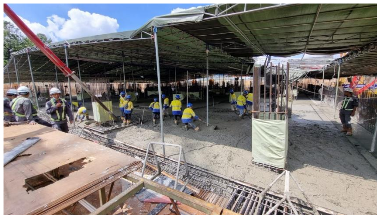
Gambar 76. Pengecoran Raft Foundation
