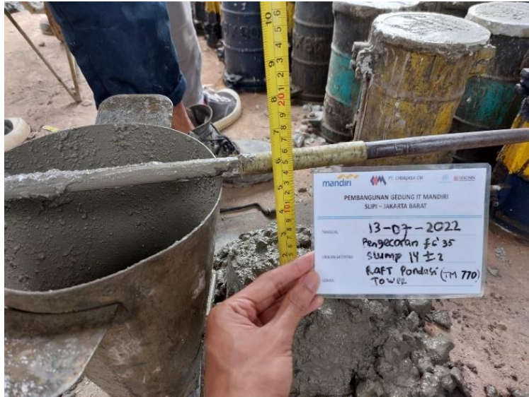
Gambar 98. Pengujian Slump Beton
