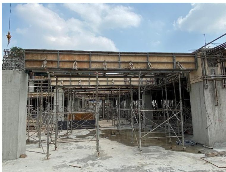
Gambar 25. Perancah ( Scaffolding ) Balok
