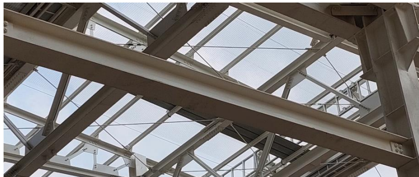
Gambar 4. 13 Balok H Beam
