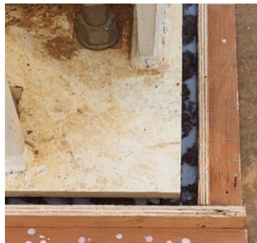
Gambar 5. 43 Bekisting in Situ
