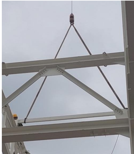
Gambar 5. 9 Proses Erection Purlin
