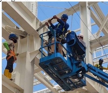
Gambar 5. 37 Proses Tightening Bolt
