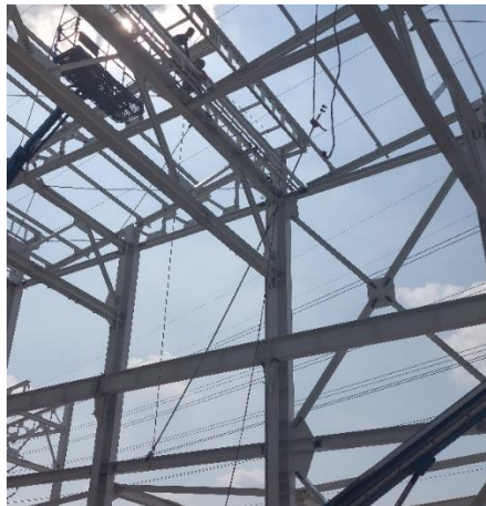
Gambar 5. 18 Proses Erection Ikatan Angin
