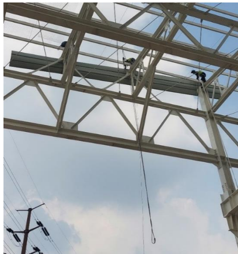
Gambar 5. 27 Proses Erection Material Atap
