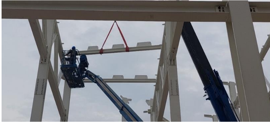
Gambar 5. 7 Proses Erection Rafters
