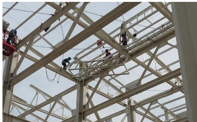
Gambar 5. 21 Proses Erection Fasad Kaca
