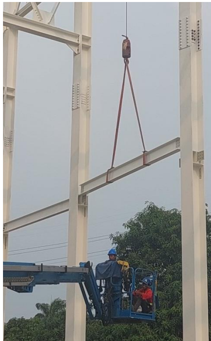
Gambar 5. 3 Proses Erection Balok
