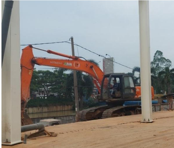
Gambar 4. 45 Back Hoe (Excavator)
