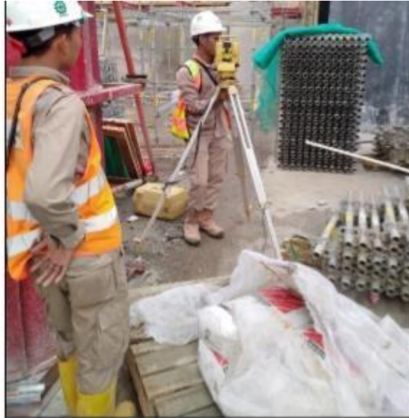
Gambar 2.27 Marking as Shearwall
