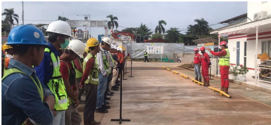
Gambar 2.6 Kegiatan safety morning talk di Proyek Cibinong City Mall Extension.
