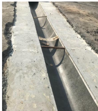
Gambar 4.20 Pemasangan flushing (talang air expansion joint)
