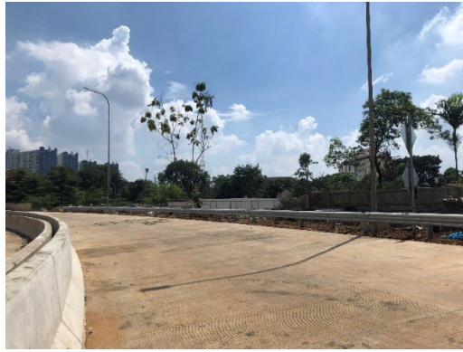
Gambar 4.3 Monitoring Guardrail dan Parapet
