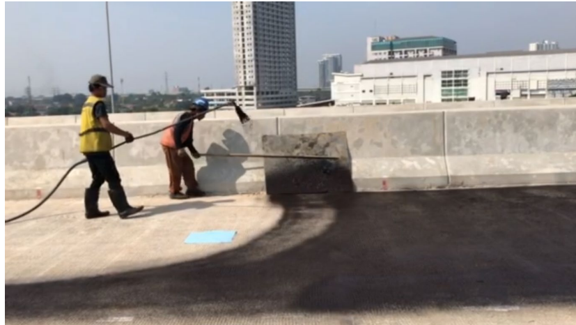
Gambar 3.27 Penghampanan Tack Coat
