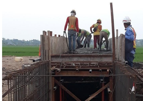
Gambar 3.27 Pengecoran Box Culvert
