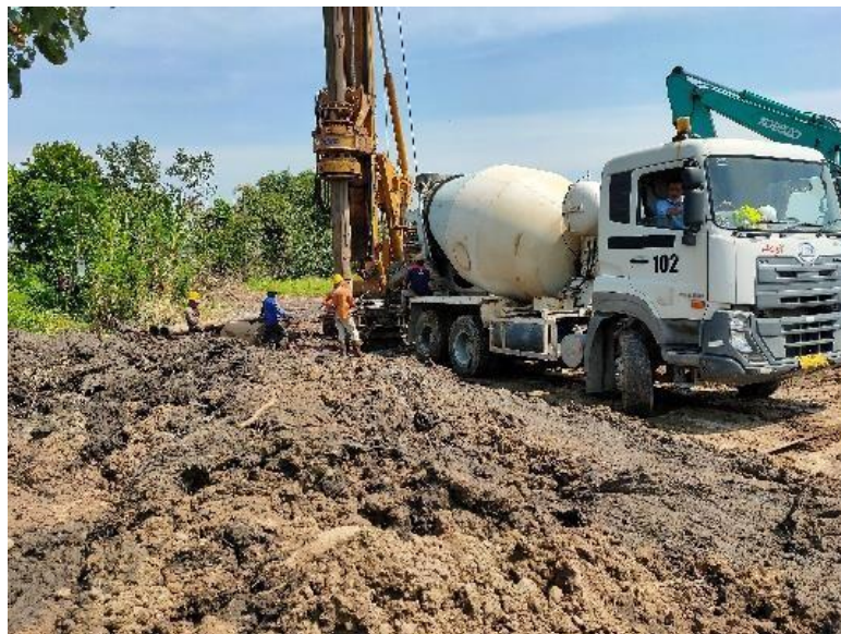
Gambar 3.20 Proses Pengecoran Bored Pile
