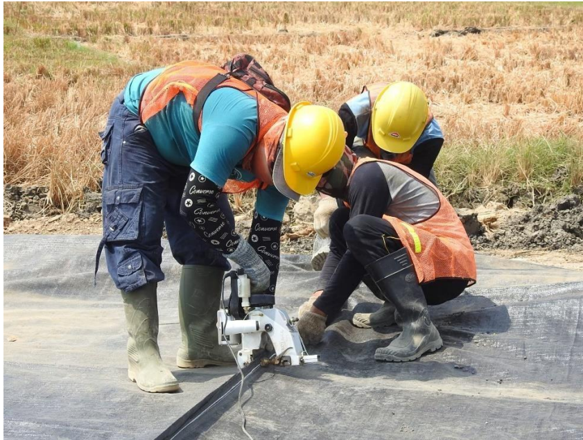
Gambar 3.12 Proses Panjaitan Geotextile Woven
