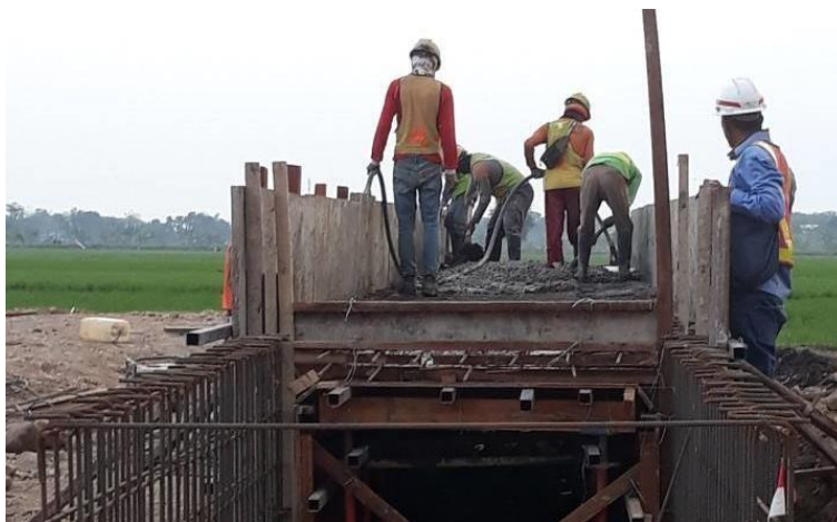
Gambar 3.35 Proses Pengecoran Dinding Underpass
